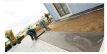
2) Attach the fabric with DuPont™ Plantex° anchor pins. For large areas requiring more than one fabric, allow for a 10 cm overlap.
